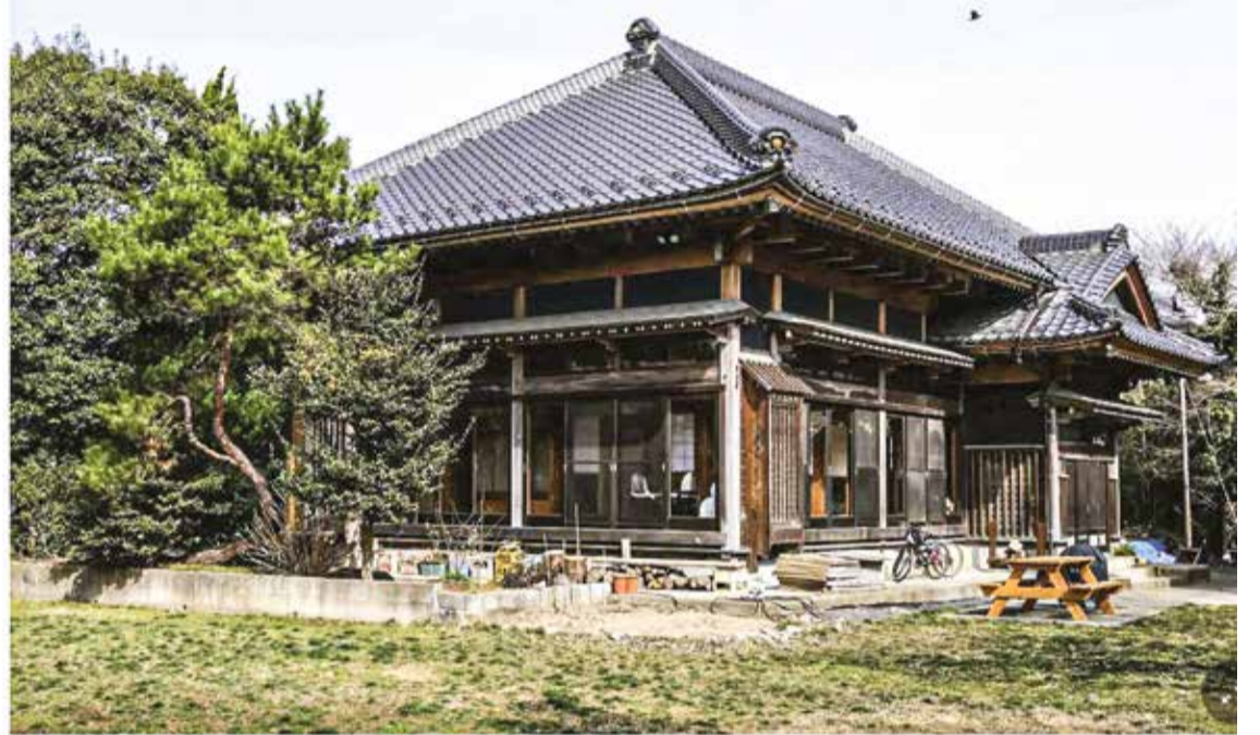
The Thursfields' house in 2019, shortly after they bought it. The house had been deserted after the previous owner's family refused to inherit it upon the owner's death. Andrew Faulk for The New York Times
